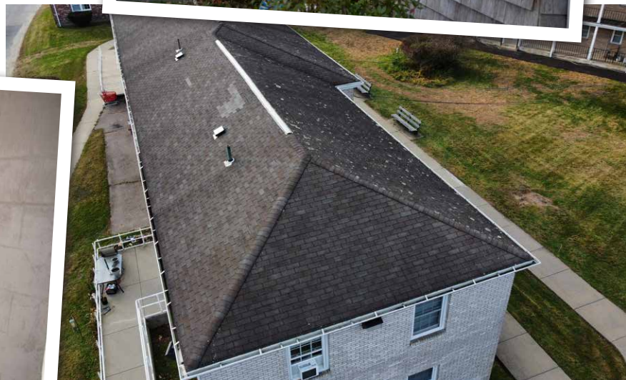
Roof replacement – Belair Heights (currently in process)
